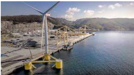
Windfloat Atlantic Project (Portugal)
